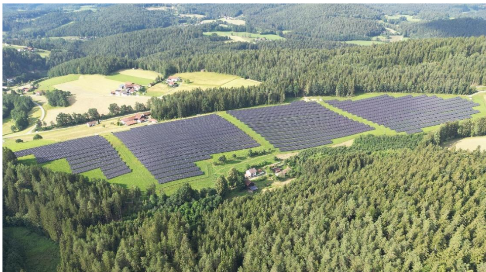
Pignet solar park near Viechtach (Germany).
